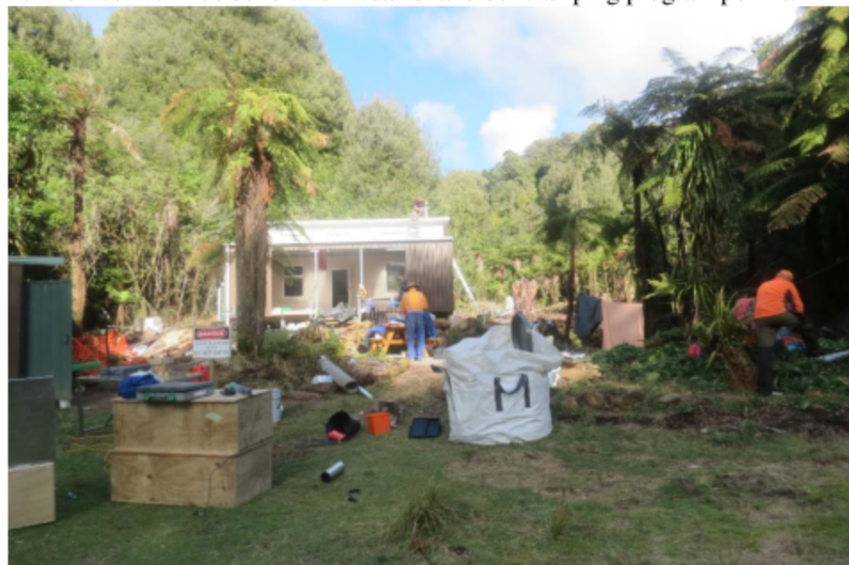
Okioki hut on the Kaimai Ridgeway track – nearly finished
